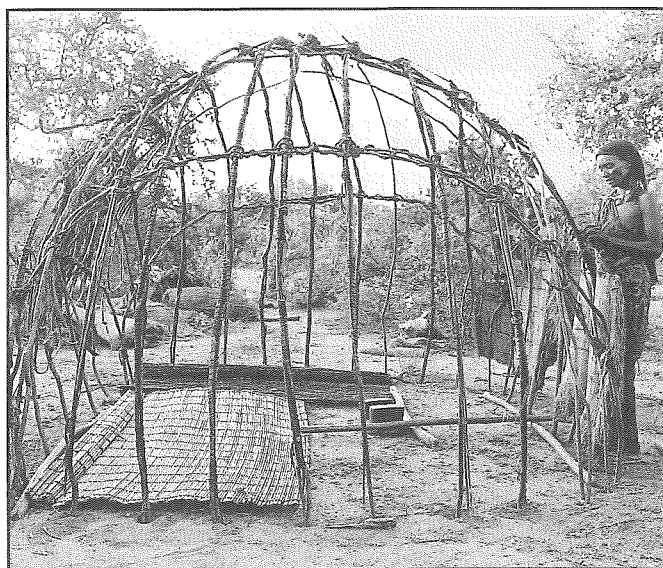
House constructing using locally harvested tree products, near the Kenya Somali border. Photo: © Oxfam
