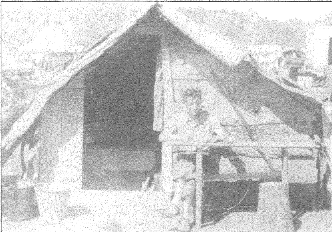
Improvised shelter at Viktring camp; roof and walls made from bark stripped from local trees Photo: Collection of Prof Uros & Mrs Roessmann
