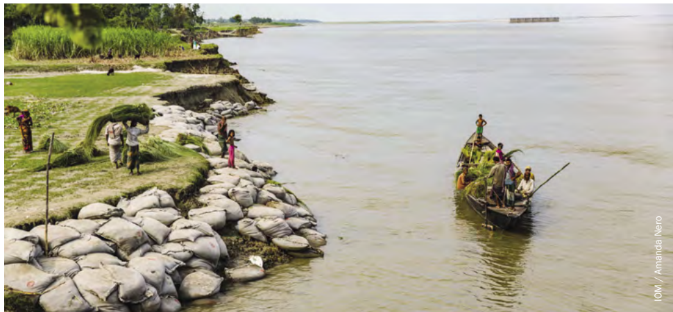
Community members in Sirajganj district in Bangladesh have worked to protect their land against river erosion, which has displaced many people several times.
