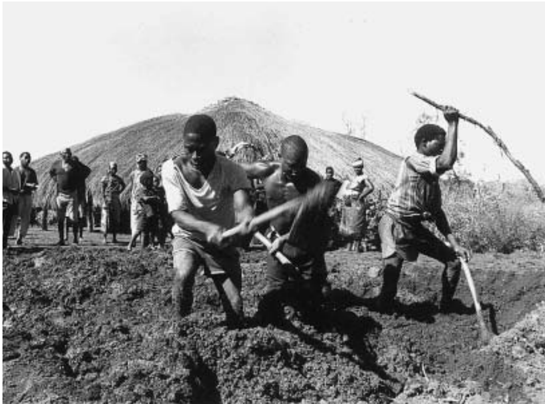
Mixing mud for walls of new community meeting house, Zambesia, Rwanda
