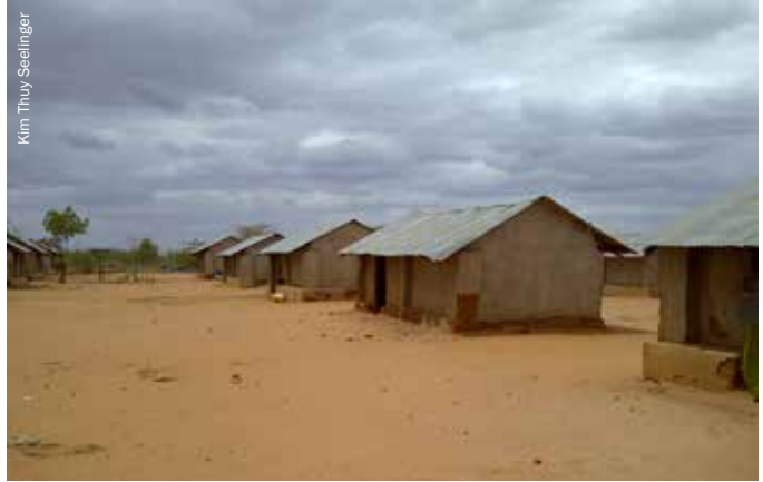
Safe Haven shelter in Dadaab refugee camp in Kenya, 2011.
