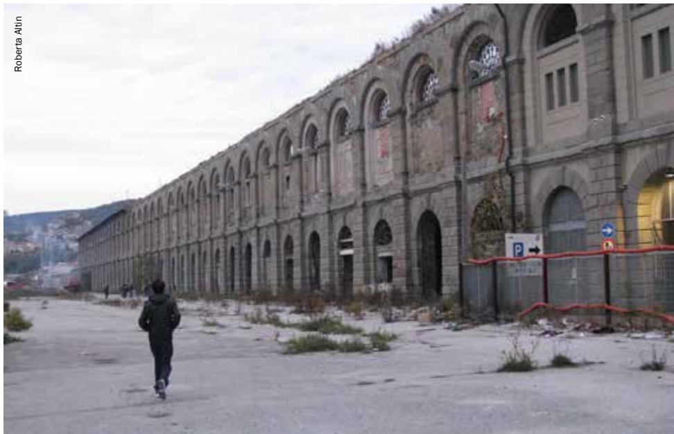
Silos, in Trieste, Italy.
