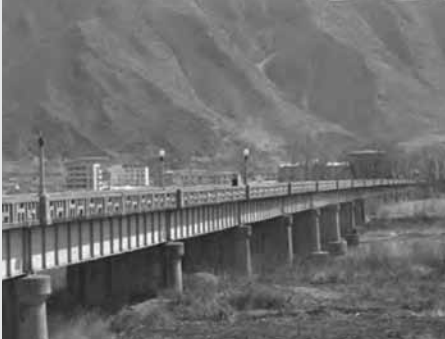
The bridge connecting Tumen in China and Namyang in North Korea, over the Tumen river.
