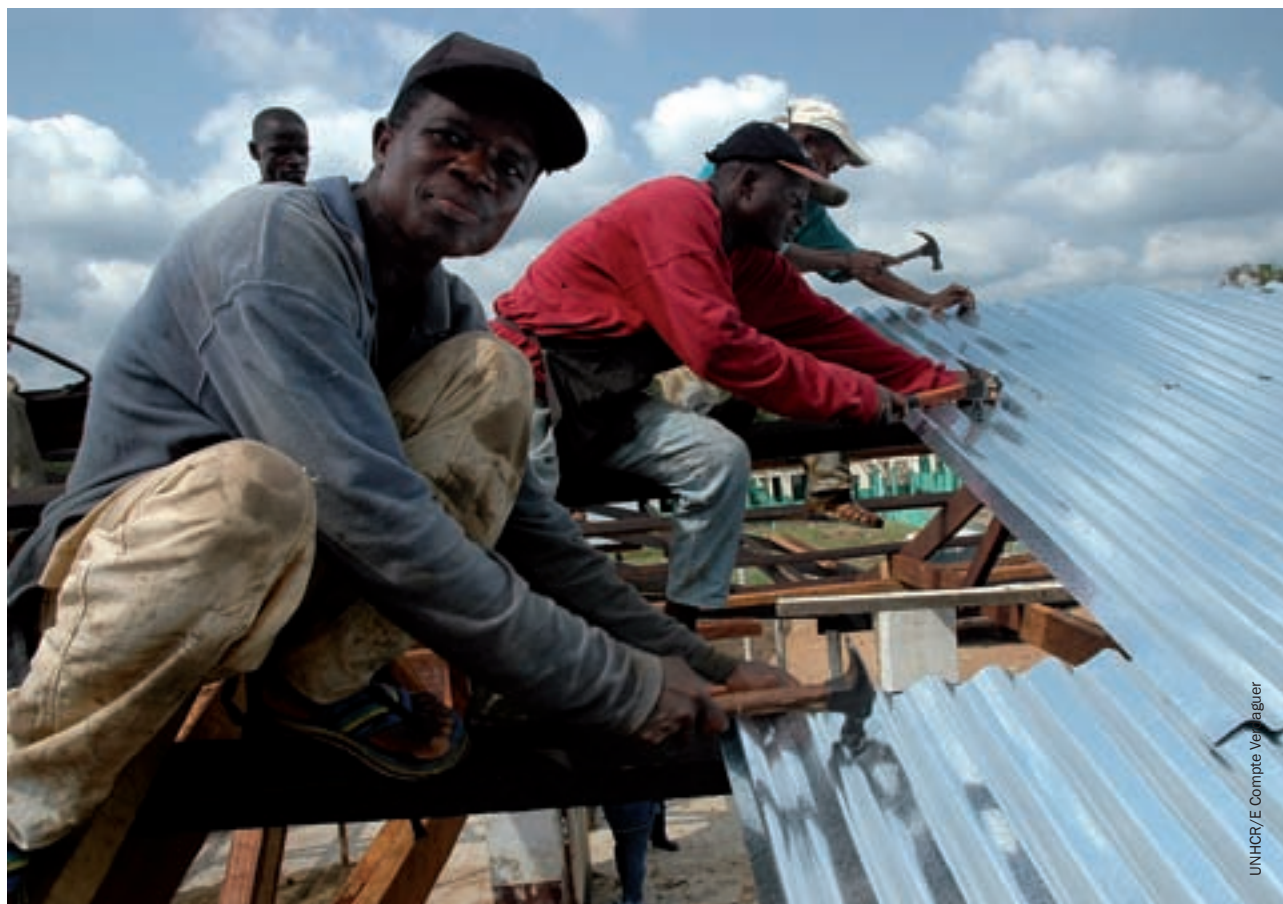
As part of UNHCR's community empowerment projects, workers build a school and pass on their construction skills to younger returnees in Gbarlatuah, Bong county, Liberia.
