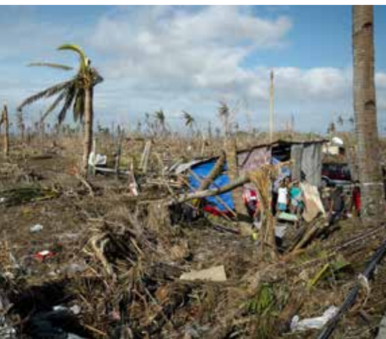
Destruction wrought by Typhoon Haiyan in the town of Tanauan in the Philippines, November 2013.
