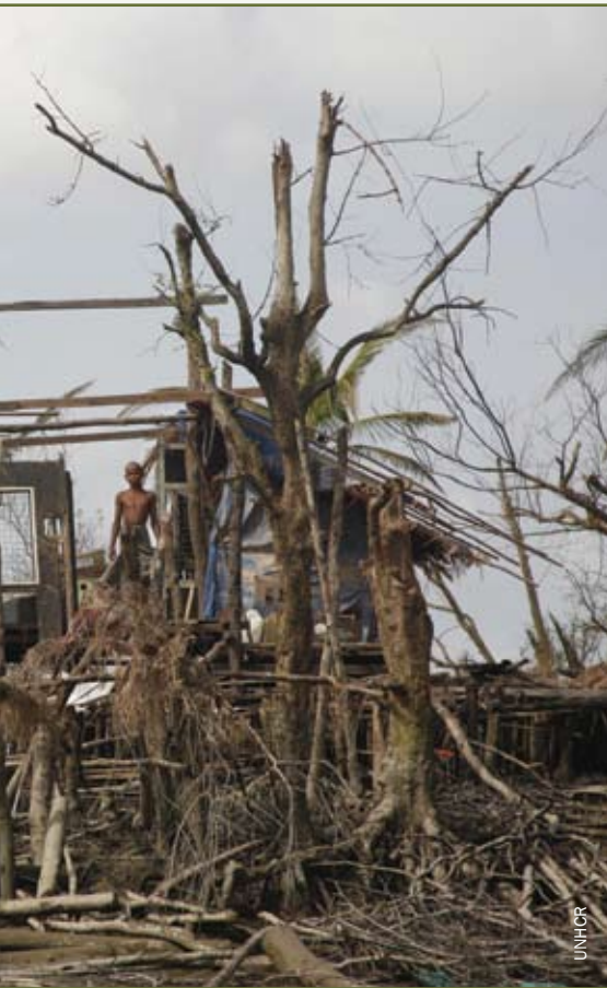
Ruins of a home destroyed by Cyclone Nargis.
