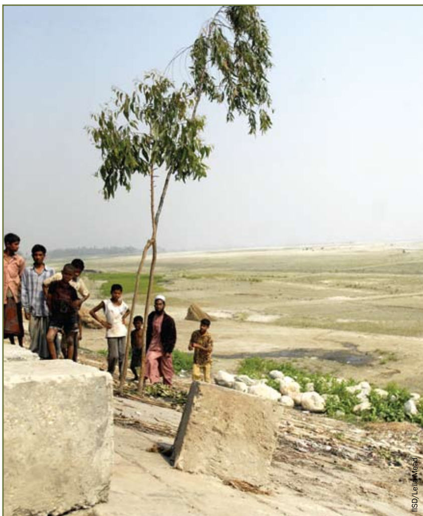
River bank protection along the Brahmaputra River, Bangladesh. 2007
