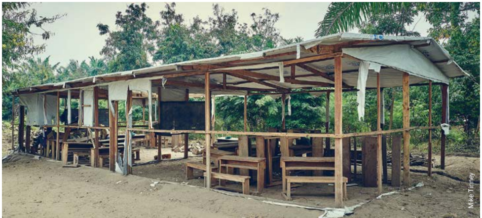
Temporary learning centre in Lusenda refugee camp, Democratic Republic of Congo, constructed in such a way that it can be easily converted in future into a permanent structure at low cost.
