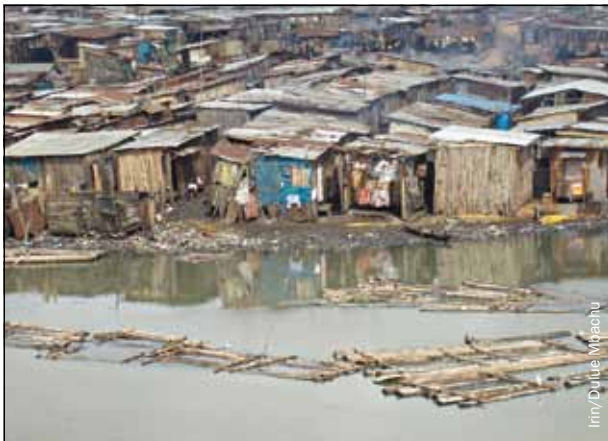
Slum housing in the Ebute Metta district of Lagos, Nigeria.
